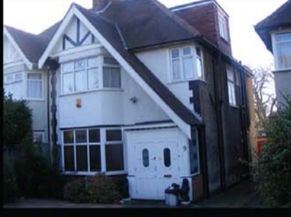
MILL HILL 4 Bedroom House £699,950
